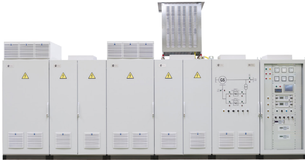
Totally redundant DECS-400 system
